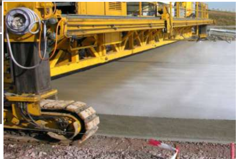
Exposed aggregate concrete (highway construction)
