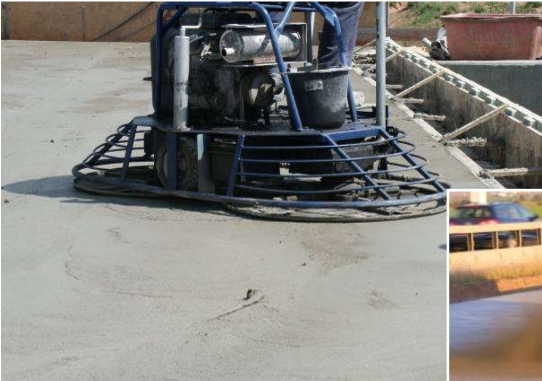
Power floating (bridge deck)
