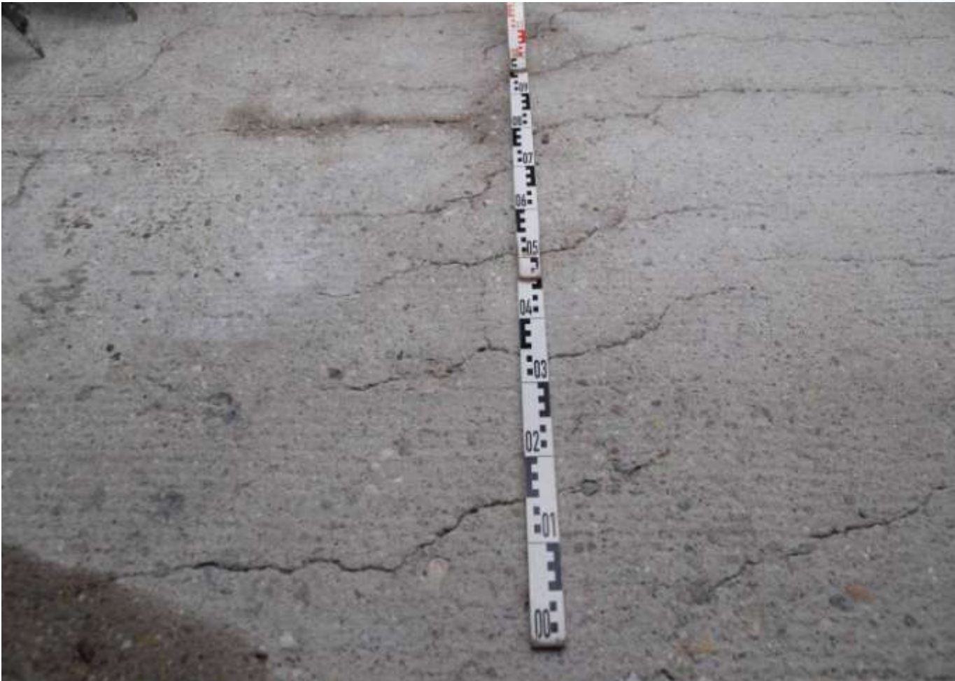
Cracked concrete floor (parking structure)
