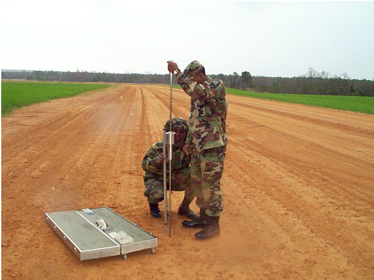
FIGURE 2 Picture of the DCP in Use
