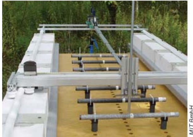
A dowel bar alignment is set up for a field validation at the testing facility.
